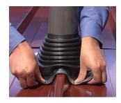
Slide the Roof Boot down over the pipe. Moisten the pipe to overcome friction and slide the Roof Boot down into position.
