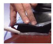
6 Finish by applying at continuous bead of silicone to the edge of the flange and smooth off.
