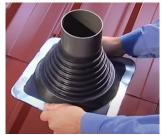
Use self drilling washered screws or sealed rivets to fasten the Roof Boot to the cladding.
