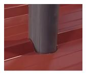
Press flange onto roof cladding and silicone. Mould to shape easy out any creases. Don't over stretch the billowed cone adjust the fit on the pipe as required. Leave some 'give' in the flexible cone to allow for minor movement.
