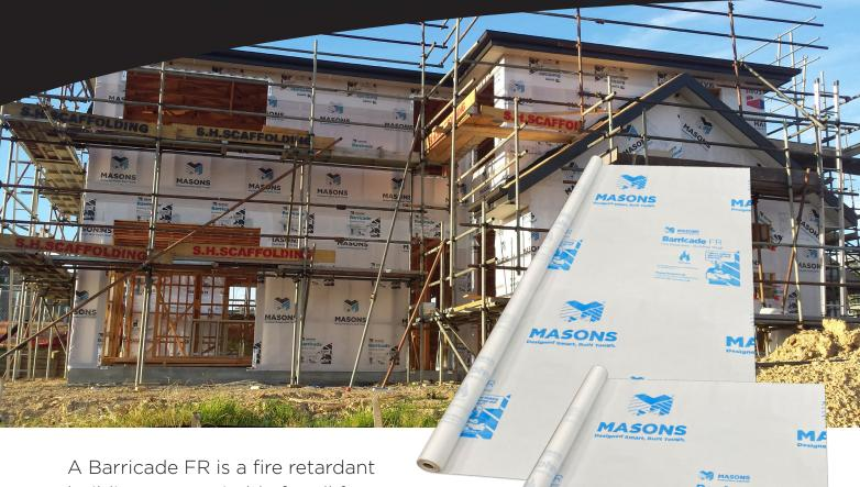
A Barricade FR is a fire retardant building wrap suitable for all frame and cladding systems with or without cavity. It is Codemark Certified.
